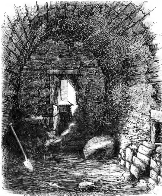
Fig. 8. Interior of the building, showing splayed window in eastern gable, recess in interior of south wall, vaulted roof, etc.
